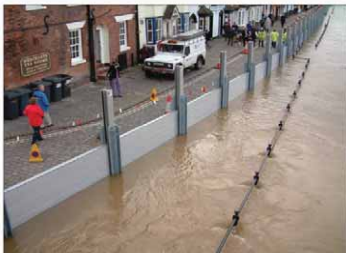
Flood defences in operation in Bewdley last summer
