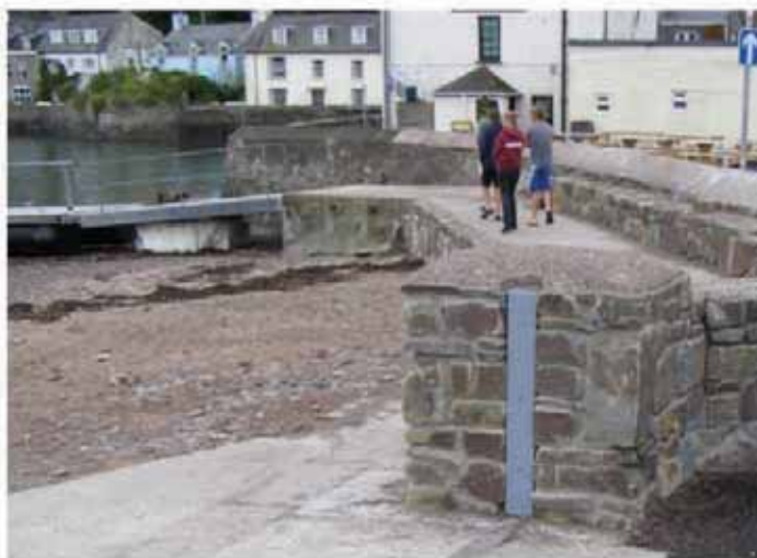
Dale harbour with the defences demounted
