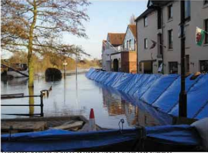
Temporary barriers in place at Upton-upon-Severn last summer
